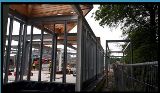
John Turner Construction – Birtenshaw School, Bolton
